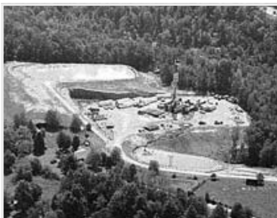
Gas well drilling pads typically cover several acres. The artificial ponds hold water (and, later, polluted water) used for fracturing. A fully-developed gas field might have one pad every few thousand feet.
